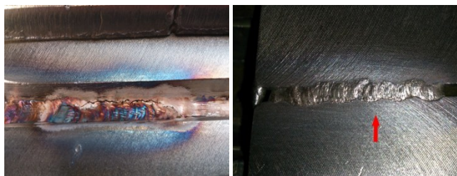
Fig. 2. View of a crack created in the joint root part (a red arrow pointing at the crack)
