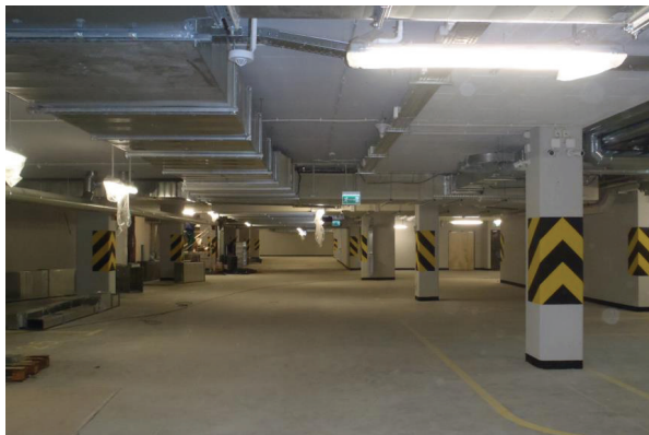
Fig. 1. View of level –1
