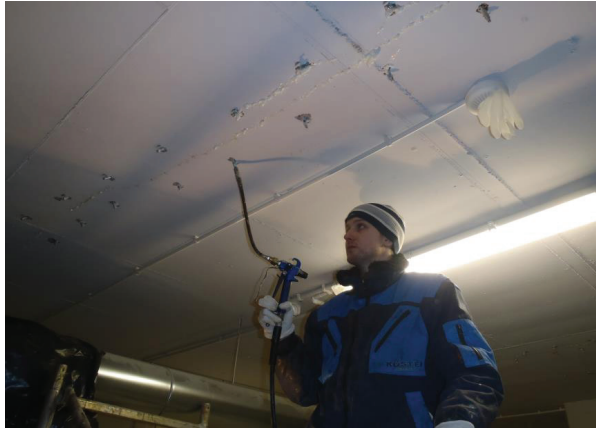
Fig. 10. Crack sealing at site 8
