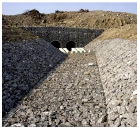
Fig. 2. The use of gabion baskets and mattresses ( http://www.ograzdamy.pl )
