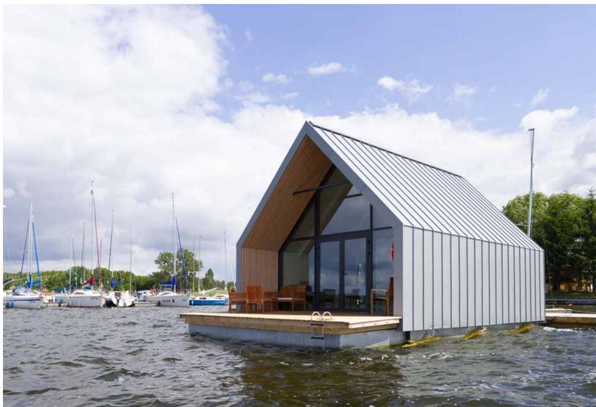
Photo 1. Completed prototype floating apartment at Lake Roś in Pisz (phot. K. Ostrowska-Wawryniuk )
