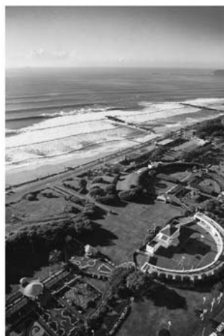
Photo 2. View of a section of ocean frontage that was to become the promenade, prior to the 1980's major upgrades. The sunken gardens and lower Marine Parade still exist with additional amenities appearing from the time of the 1930's development
