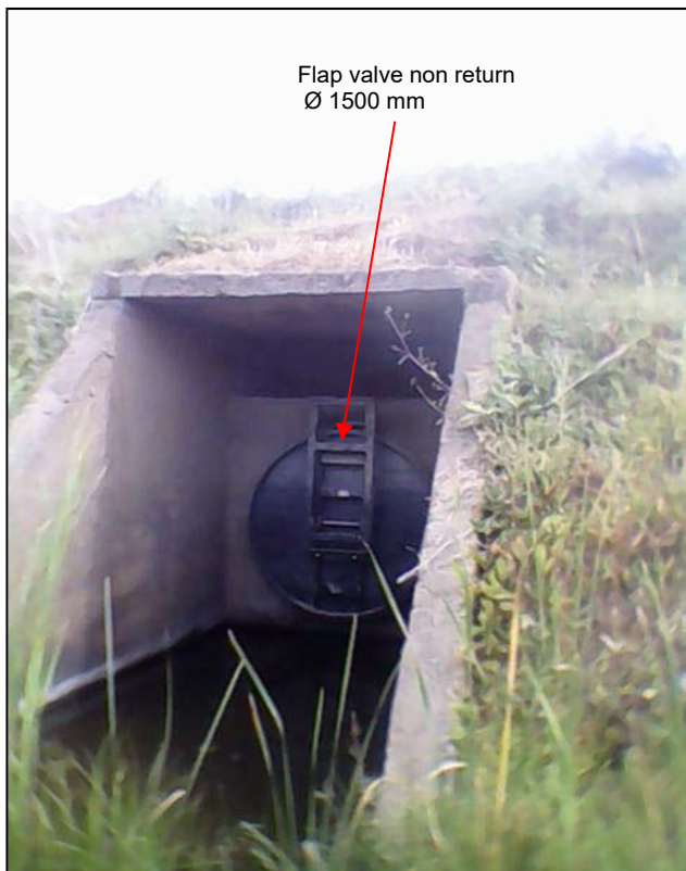
Photo 1. Downstream rejection structure of the canal towards wadi El Kebir (phot. F. Sennaoui)
