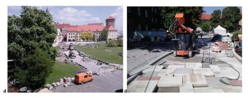
Fig. 1. Fragment of the photographic documentation of refurbishment work performed on the Outer Courtyard at Wawel Castle: (a) view of the bottom of the excavation trench; (b) uncovering of archaeological artefacts; (c) view of the aggregate subbase course being laid; (d) wearing course out of sandstone tiles, source: original photographic documentation.
