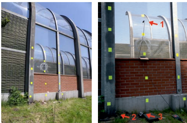
Fig. 1. The investigated noise barrier and distribution of measurement points.
