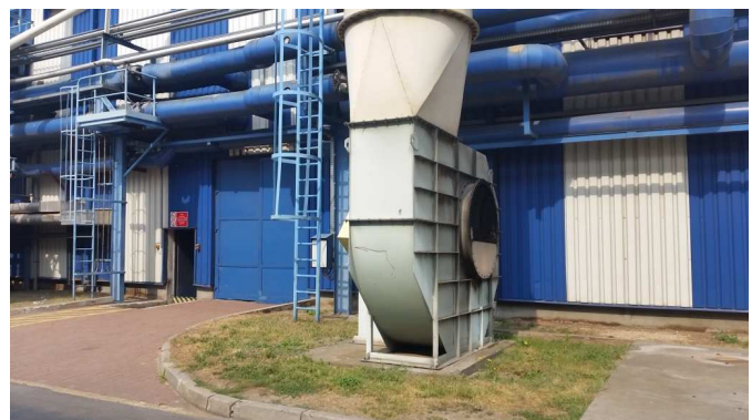
Fig. 8. Source Z3 (industrial fan) – flow Q = 120\,000\text{ m}^3/\text{h} , diameter 1.3 m, frequency range 110–120 Hz.
