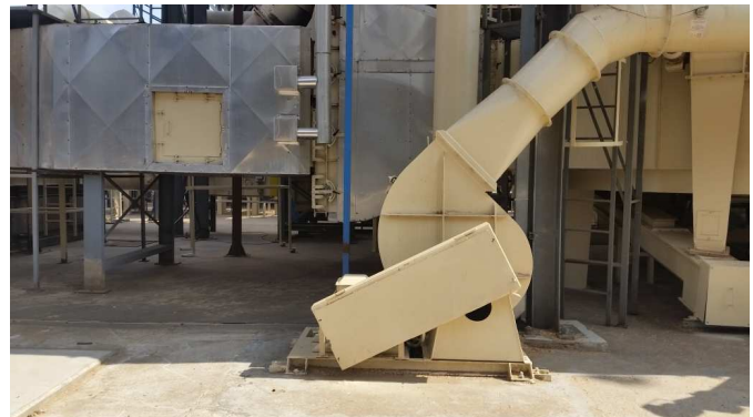
Fig. 6. Source Z2 (industrial fan) – flow Q = 14\,000\text{ m}^3/\text{h} , diameter 1 m, frequency range 230–250 Hz.
