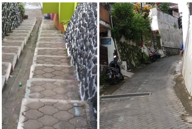
Photo 6. Paving block on sloped surfaces in the study area (phot. L. Sedyowati)
