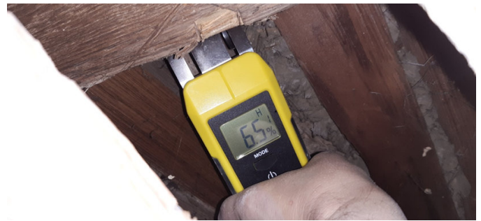
Fig. 11. Moisture content measurement of ceiling beams – test hole no. 2
