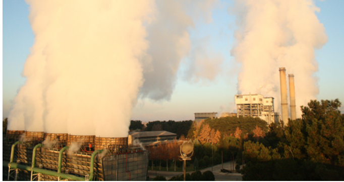
Fig. 1. Wet tower of ITPP and their output plume
