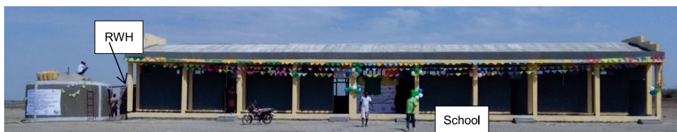
Fig. 4. Roof water harvesting (RWH) water tank and its water source – the school at Dababuraburi (phot.: M.C. Shumie)
