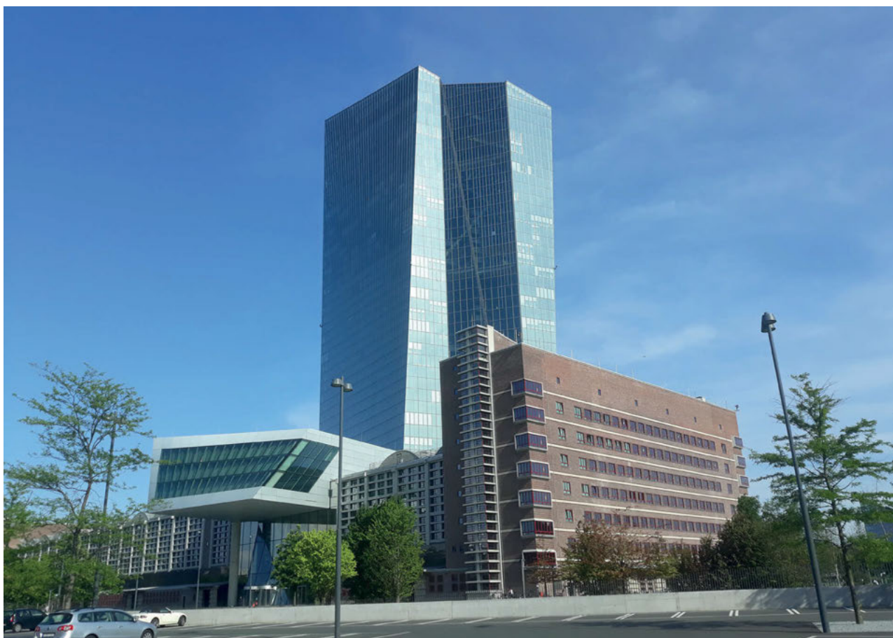
III. 5. The ECB complex as seen from the street. Photo by M. Gyurkovich.
