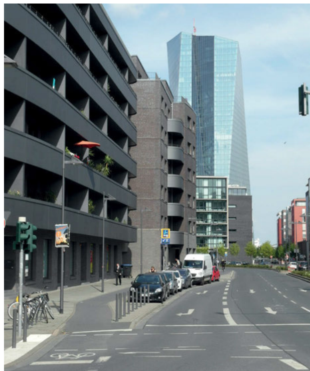
Ill. 7. The ECB as the urban dominant of the immediate neighbourhood. Photo by Z. Macri
