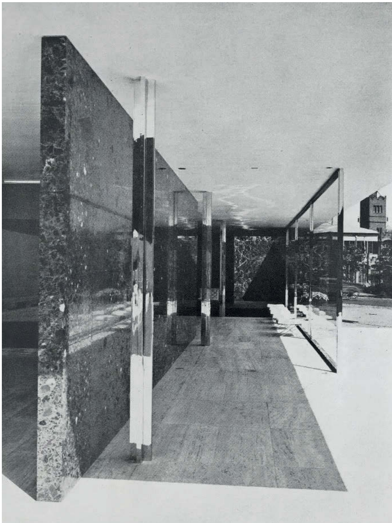
III. 2. L. Mies van der Rohe, the front part of the German pavilion in Barcelona, 1929. Green marble wall and pillars clad with polished steel. Photo by Berliner Bild-Bericht.
