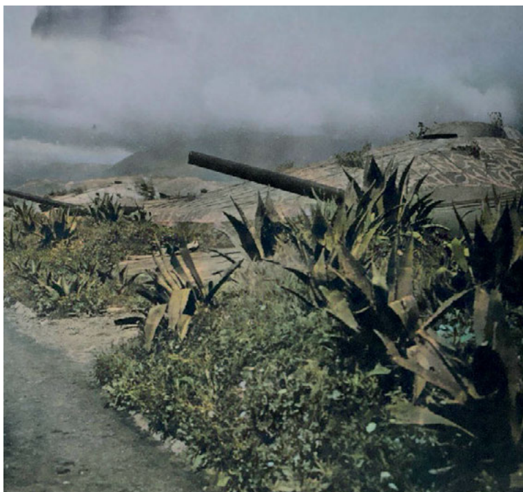
Ill. 9. Archival photograph of Caballa coastal battery (Kotor, Montenegro), colorized. Well-visible combination of two-tone camouflage painting, live vegetation found locally, and supplemental masking with cut branches around the observation post's armored cupola. Authors' own work based on original photo, Österreichisches Staatsarchiv — Kriegsarchiv, Wien, file ref. AT-OeStA/KA BS I WK Fronten Serbien, 2499.
