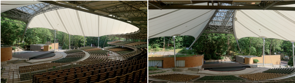
Fig. 1. The Forest Opera membrane hanging roof in Sopot, Poland – co-designed by the authors
