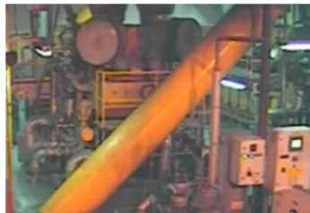
(b) t = 12 s CCTV picture
