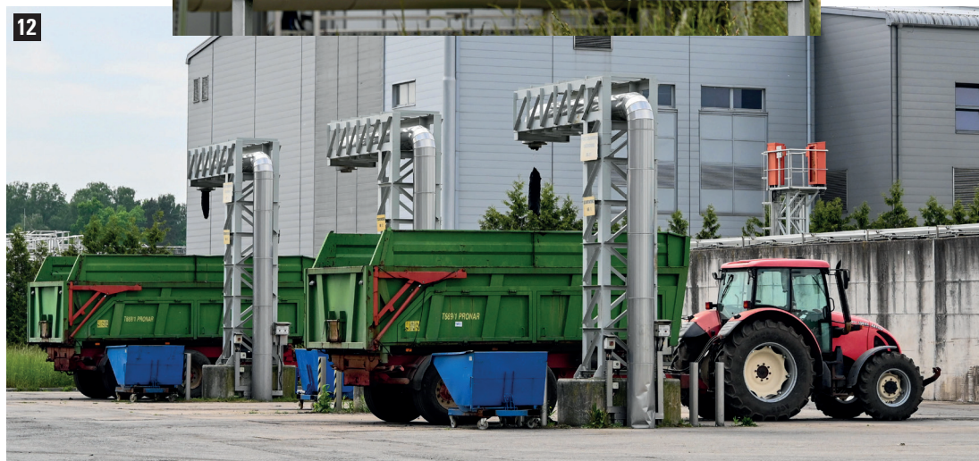
Photo 12 Stabilized sludge collection stations (operated during annual reviews of the Thermal Sludge Processing Station)
