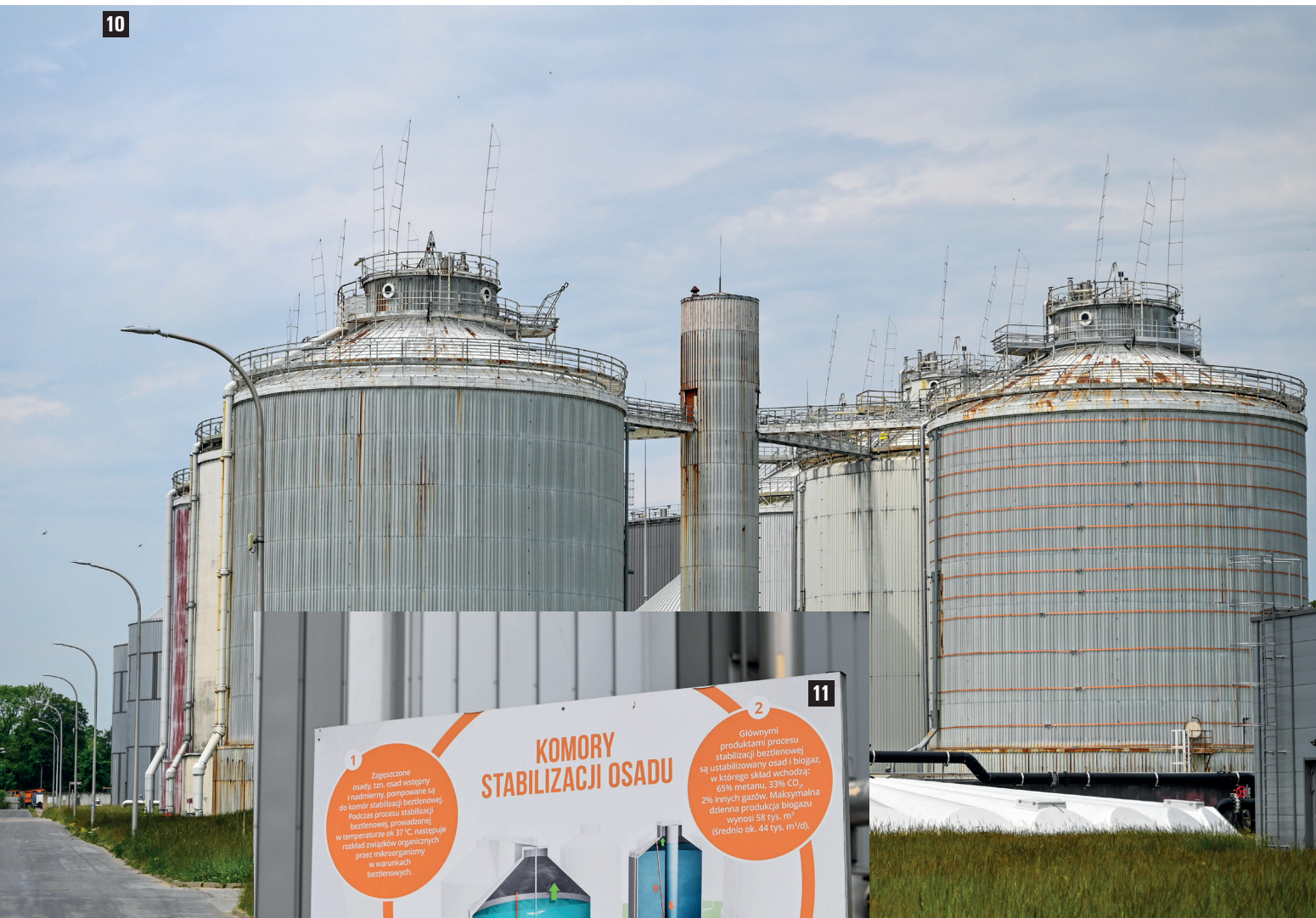
Photo 10 Sludge fermentation tanks ("digesters")
