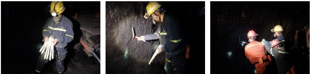
(a) Installation of end anchored and full-length anchored bolts
