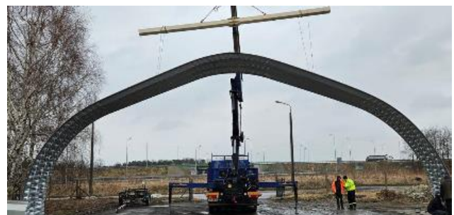
Fig.7. Assembly of group of UBM panels.
