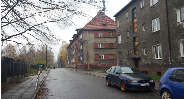
Fig. 6. View of the street along which the field measurement line P1-P6 was stabilised. Building A is visible in the background
