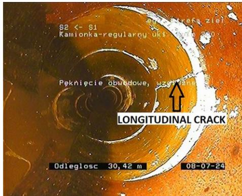
Fig.1. Example of a longitudinal crack
