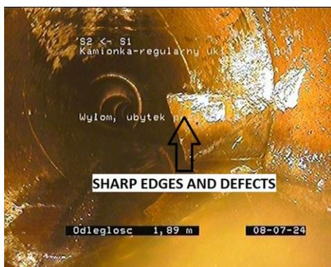
Fig.3. Example of sharp edges and defects
