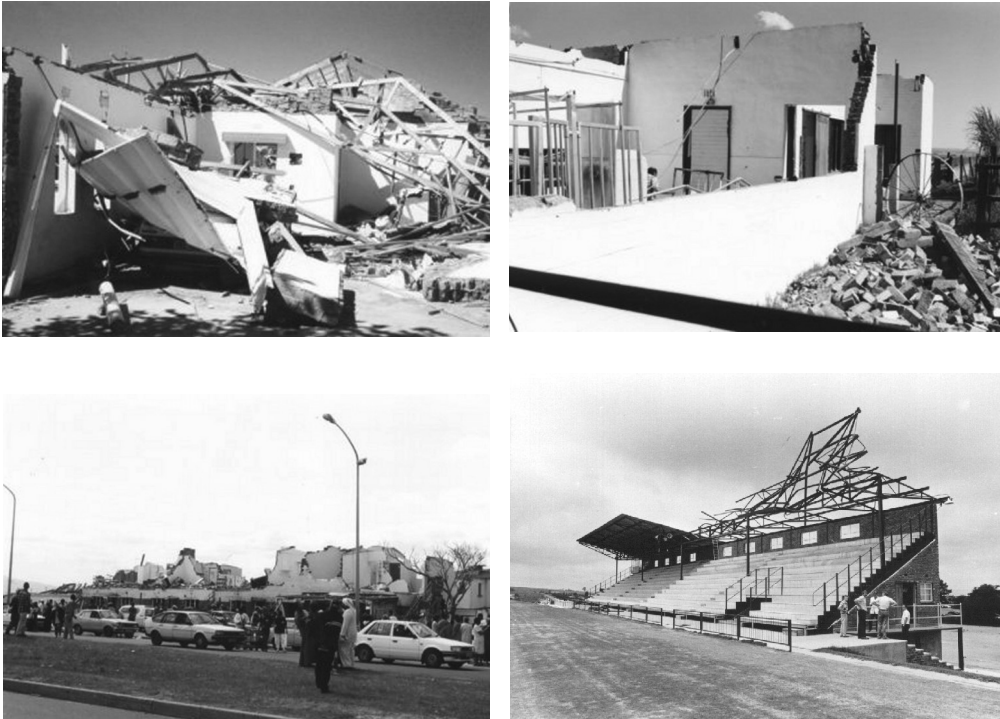
Fig. 20. Examples of serious damage in South Africa.
