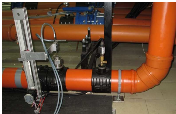
Fig. 6. The way of installing the system for traversing the measurement space and the Pitot tube.
