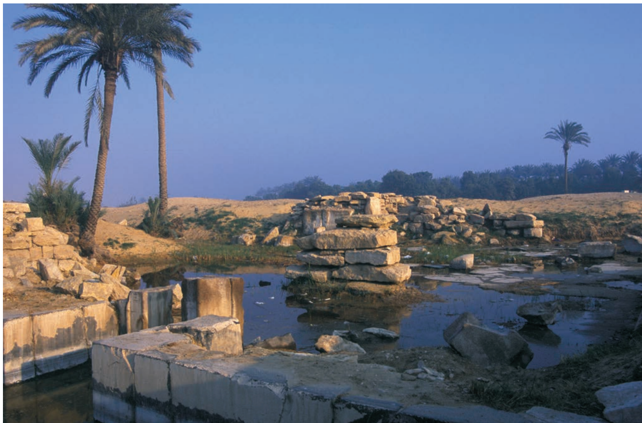
Fig. 5. Valley temple of Sahura in Abusir flooded during the rise of the water table caused by the filling of the irrigation channels (M. Bárta, Archive of the Czech Institute of Egyptology).
