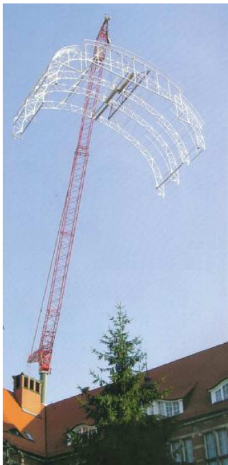
Fig. 19. Transferring glazed roof framework from the assembly site onto the Hevelius Courtyard (CYWIŃSKI, 2012).
