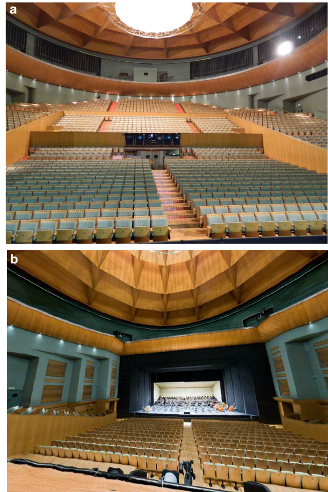
Fig. 1. The Maestranza Theatre: a) view of the hall from the stage with the absorbing cylinders deployed on the drum cover; b) view of the orchestra shell with the musician positions.
