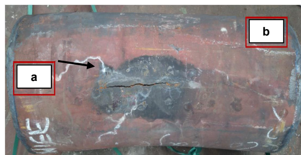
Fig. 2. (a, b) The areas from which samples were taken for mechanical properties testing: a) damaged area, b) not damaged area
