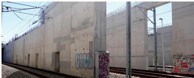
Fig. 3. Tunnel walls at the construction stage at time of analysis
