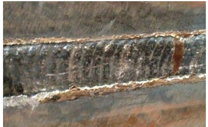
Fig. 3. A view of the face of weld made by 722 method in PF /g55 mm position
