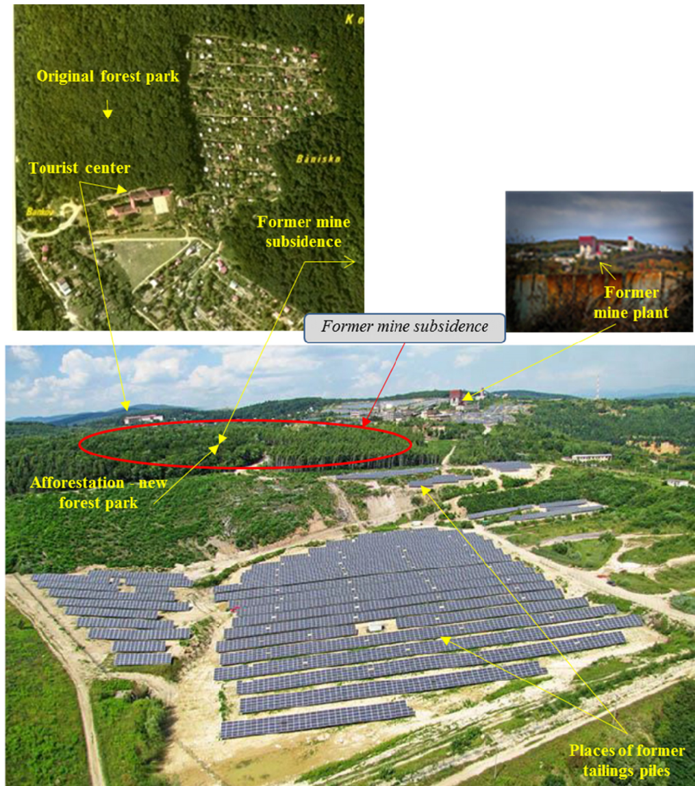
Fig. 8. Mine subsidence and surrounding (Košice-Bankov) after reclamation; panoramic view: summer 2016. Solar collectors in the places of the former tailings piles; afforestation (in the background) in the place of the former mine subsidence
