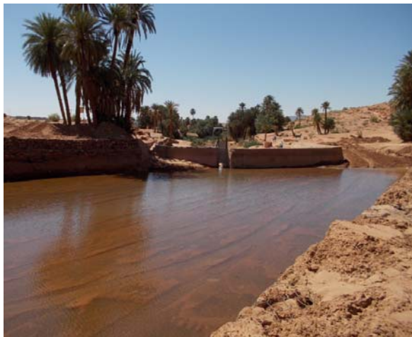
Photo 5. The ancestral Tiout dam is filled with water leaks (phot. B. Remini)
