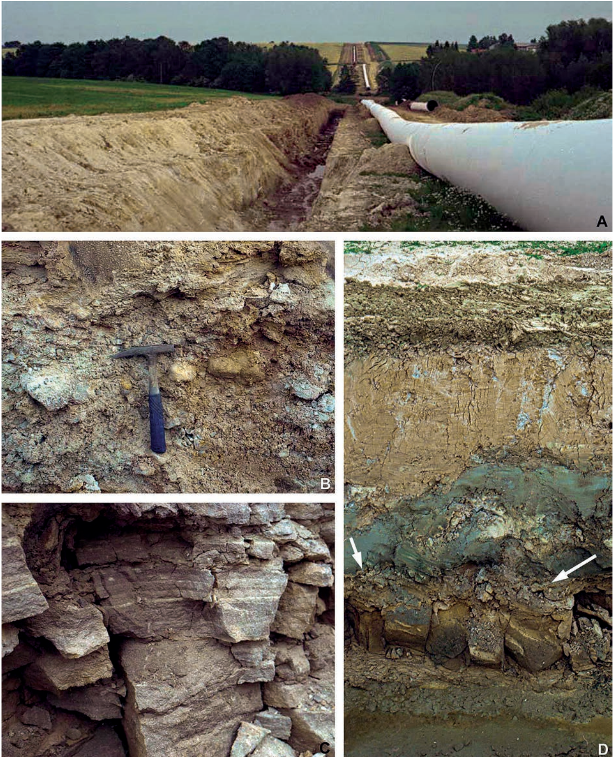
Text-fig. 4. Field aspects during excavations for the OPAL pipeline in the Dittmannsdorf area in 2011. A – trench of the OPAL pipeline north of Niederschöna (view towards the northeast). In the foreground, fluvial strata of the Niederschöna Formation are exposed; in the background (behind the wooded belt), Proterozoic gneiss crops out capped by a red-weathered palaeosol (caused by pre-Cenomanian “Rotlehm-Verwitterung”). B – lower part of the fluvial Niederschöna Formation consisting of coarse-grained pebbly sandstones with conglomerate lenses (so-called “Grundschotter”). C – cross-bedded fluvial sandstones of the Niederschöna Formation up-section of the Grundschotter. D – detail of the OPAL pipeline trench 2.5 km northwest of Haida showing the contact of the Niederschöna Formation below and a basal greensand of the Mobschatz Formation above (arrows); the uppermost part of the section is composed of Quaternary loess
