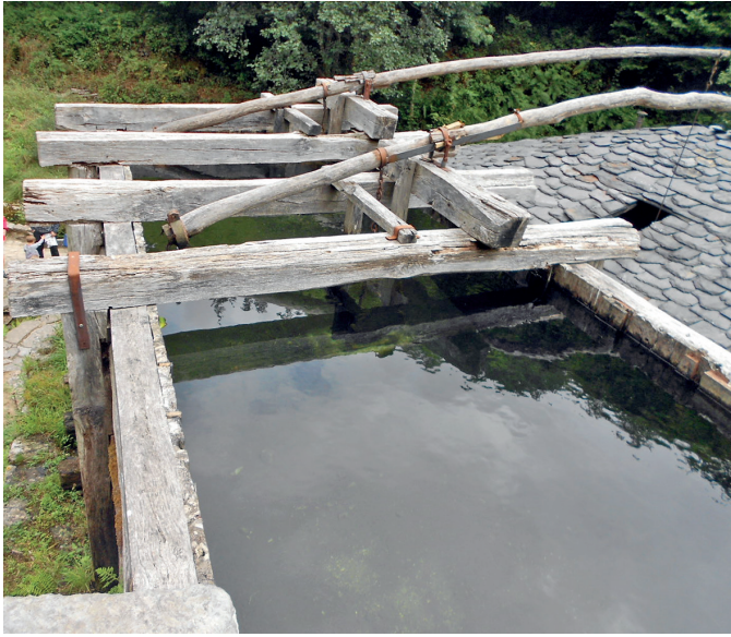
Fig. 3. Detail of the two pulls for the valves that fill the two vertical conduits
