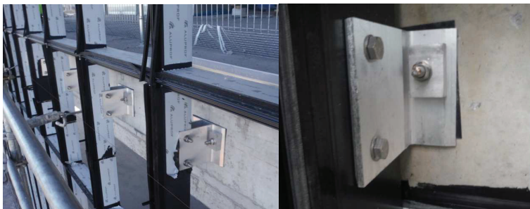
Fig. 1. Mullion-transom wall system – aluminium profiles and brackets
