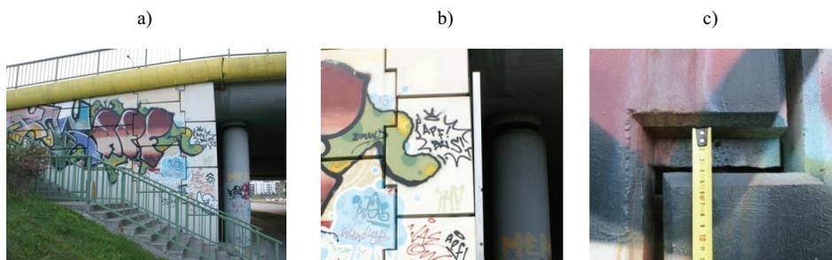
Fig. 11. Examples of deformation of the reinforced soil abutment in the case of the abutment P1: a) side view of the abutment with the curvature of the front wall face; b) detail - the deviation of the front prefabricated facing panels; c) detail - the relative displacement of the prefabricated facing panels
