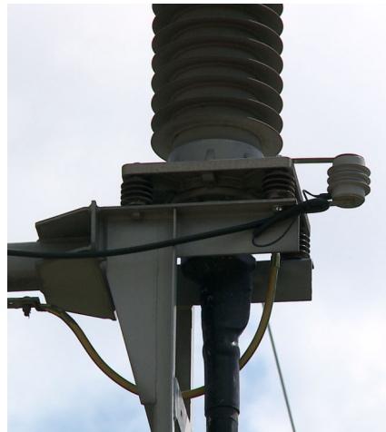
Fig. 2. Mounting method of a UHF sensor on the cable head.
