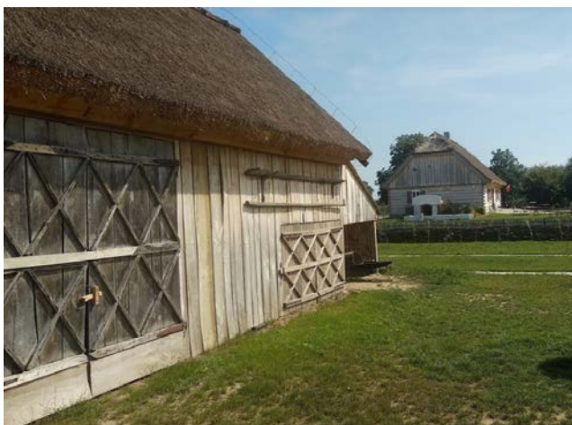
Photo 1. Traditional 'Olender' home with a lower level utility room that is periodically flooded and a boat used for travel and evacuation purposes; Antique building museum in Wiączemin Polski (Pol. Skansen Osadnictwa Nadwiślańskiego) (photo R. Mazur)
