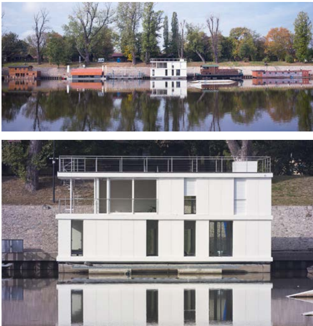
Photo 5. Floating house in the Czerniakowski Port, Warsaw – designed by Mai Bui Ngoc and Rafał Mazur: top – landscape context, bottom – zoom (phot. M. Czerski )
