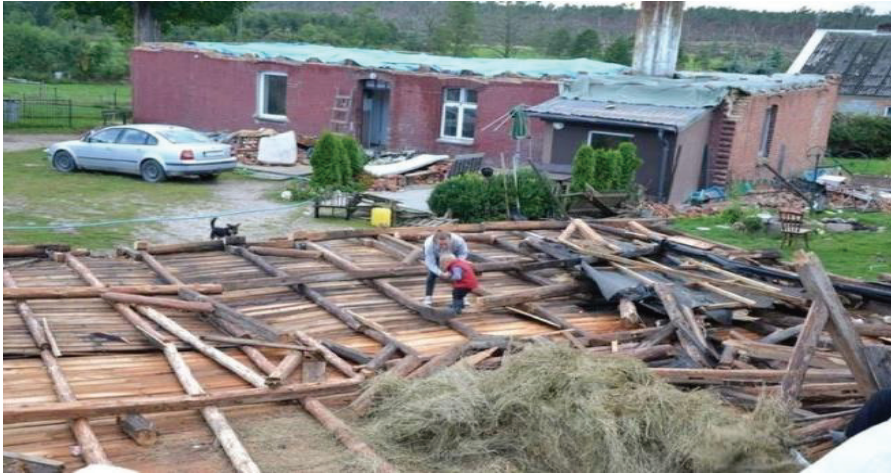
Fig. 1. The house with the roof blown-off (Source: [6])
