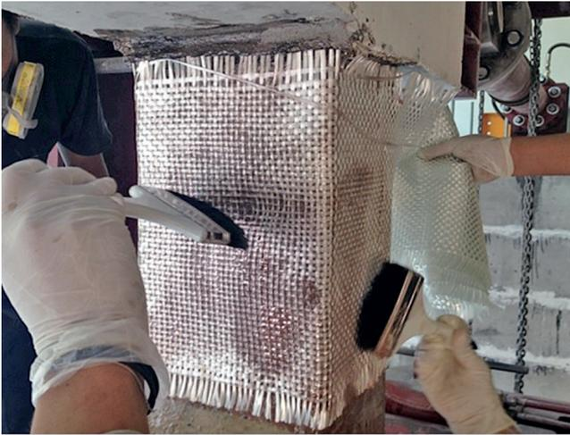
Fig. 7. Installation of the glass fiber sheet
