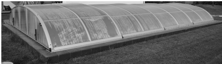
Figure 1: View of swimming pool with retractable swimming pool enclosure [7].
