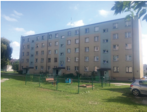
Fig. 1. Residential building (Kielce-Szczecin technology) Jędrzejów, st. B. Krzywoustego 8, 22.09.2019
