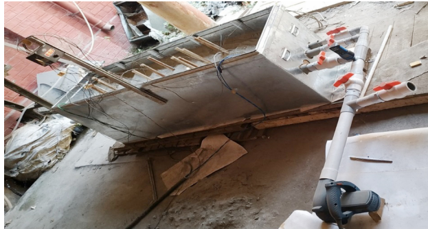
Figure 2: Photograph of the EAHE test rig.
