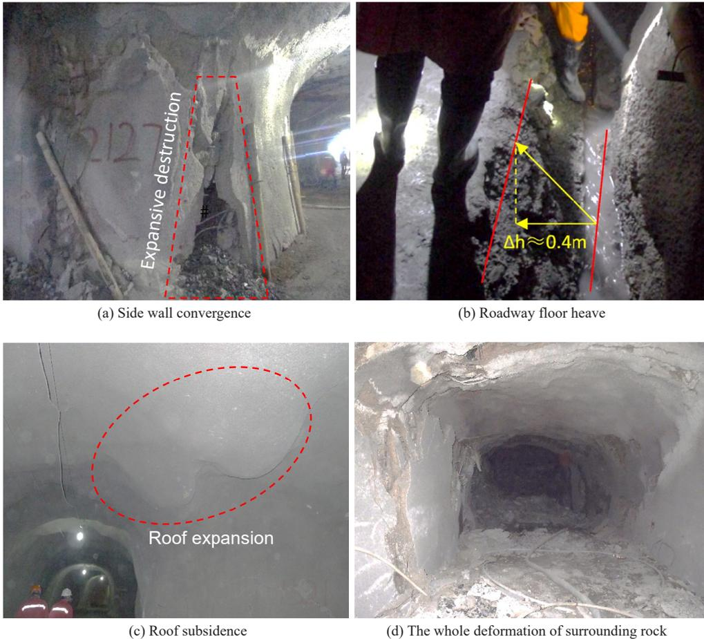
Fig. 3. Different destruction modes of expansive soft rock roadway during the rainy season
