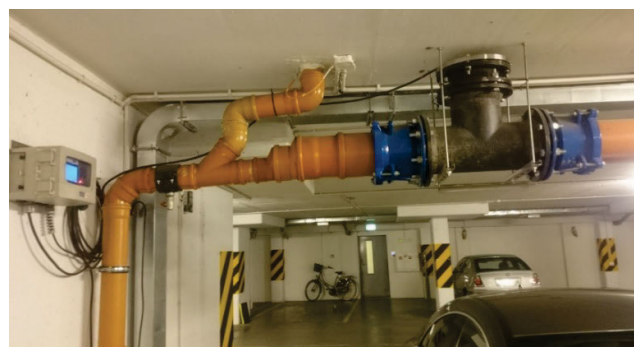
Photo 2. Measurement of stormwater flow rate and the sampling point (phot.: Archive of the Institute of Environmental Engineering and Building Installations)
