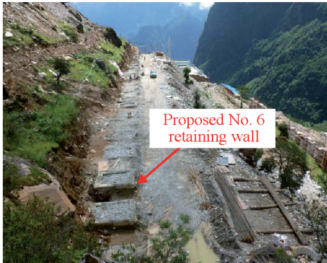
Fig. 4. Backfill of anti-slide pile holes with pebbles
