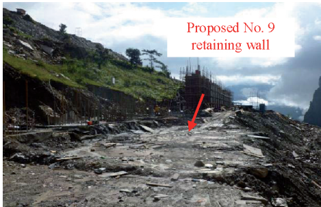
Fig. 2. Photo of No. 9 retaining wall at the leading edge of the landslide Fig. 3. Collapsed slope inside No. 9 retaining wall
