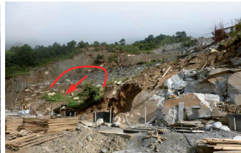
Fig. 2. Photo of No. 9 retaining wall at the leading edge of the landslide Fig. 3. Collapsed slope inside No. 9 retaining wall
