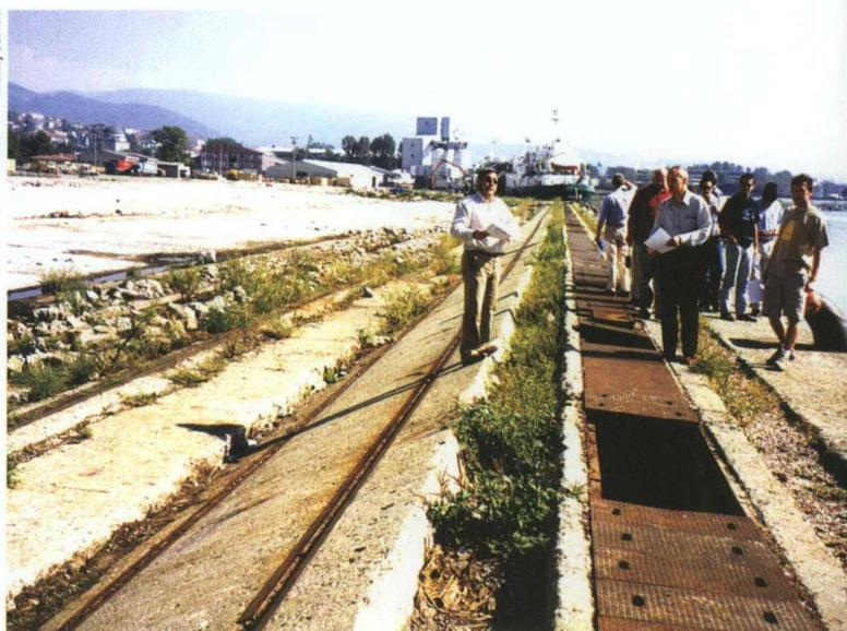
**Damaged and shifted quay-wall at the port of Derince (Turkey) caused by soil liquefaction**
