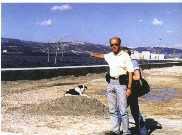
**Here a restaurant on the coastline of the Sea of Marmara slipped into the sea as a result of soil liquefaction. Emerging from the water are the tips of lamp posts which once lit the road leading to the restaurant before the earthquake struck**
