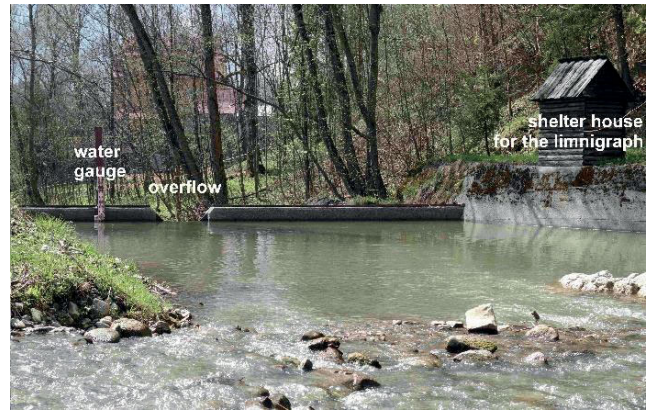
Fig. 2. The measuring cross-section with a dam on the Biała Woda stream; source: own elaboration (photo: A. Jaguś)
