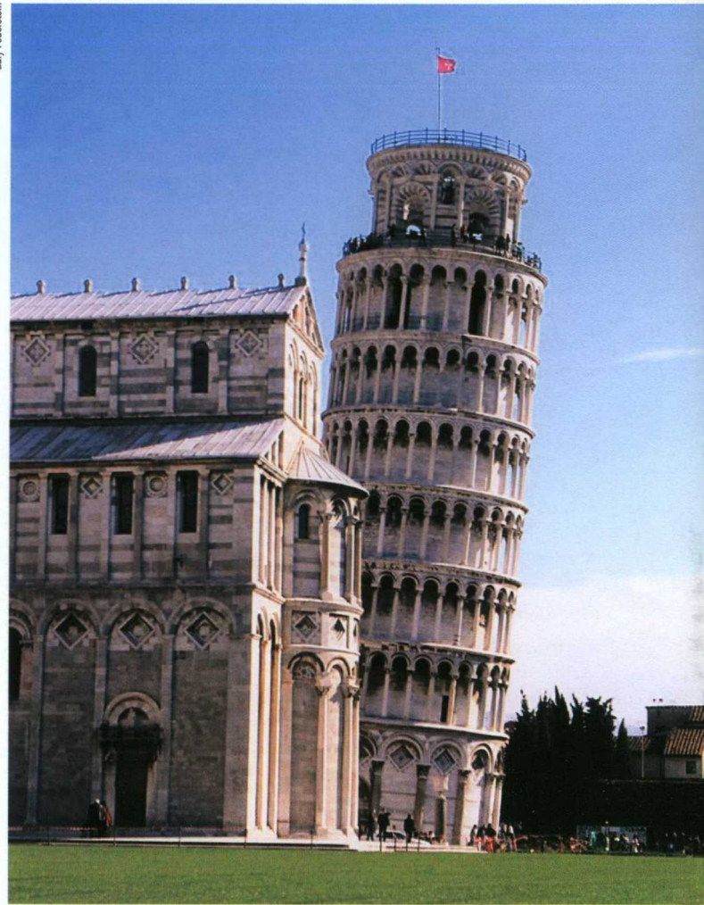
The famous leaning tower of Pisa is a perfect example of how subsoil strain can affect buildings
